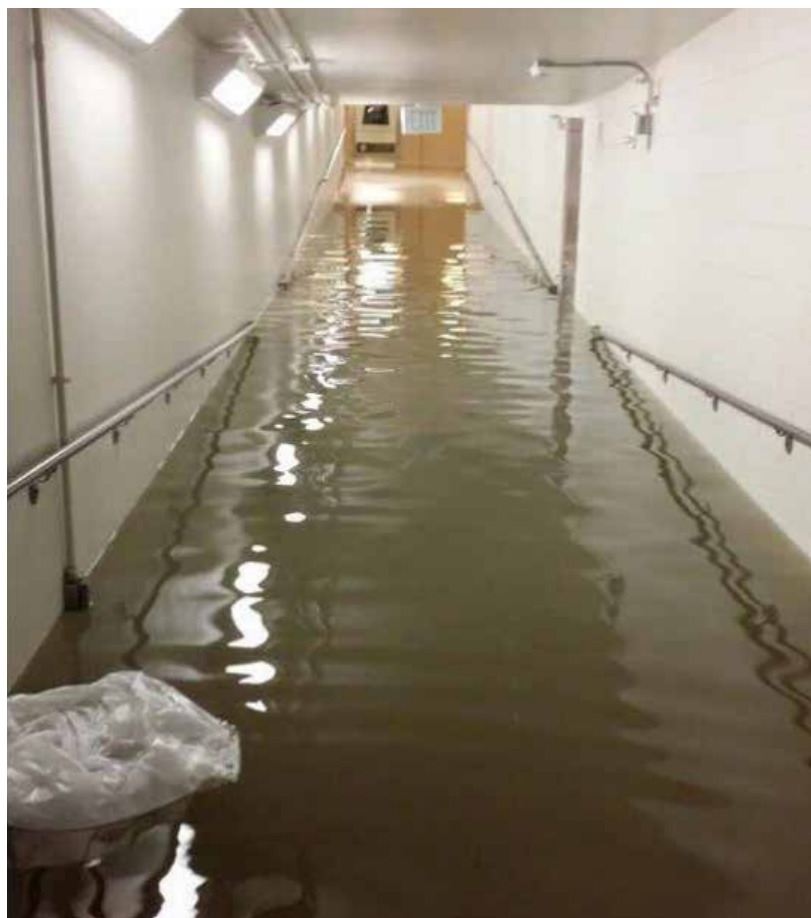
A late May storm caused flooding in a tunnel leading to the Jury Plaza - and flooded out the hotel that was to host the conference.
